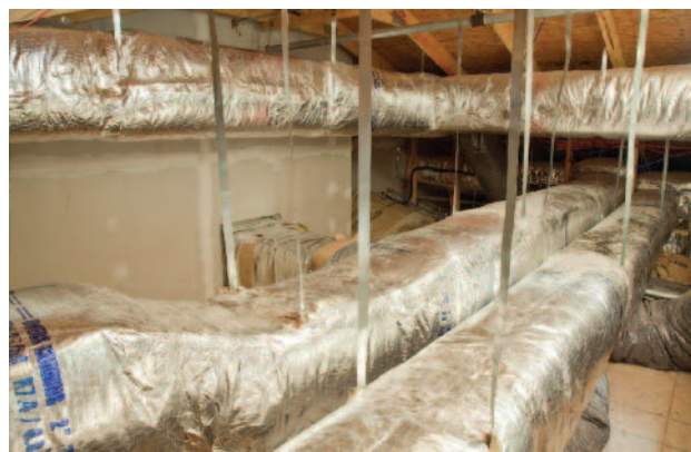
Figure 5: Cottage 6B, Glass Fiber Insulated Sheet Metal Ductwork Installation
