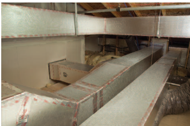
Figure 4: Cottage 6A, Kingspan KoolDuct® System Ductwork Installation
