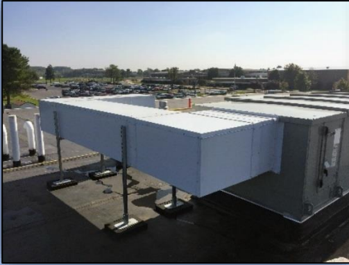
Central Dauphin School District Administration Building, Harrisburg PA
